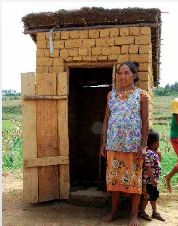
ABOVE LEFT: A FLY-PROOF LATRINE USING LOCAL MATERIALS AND BUILT AFTER TRIGGERING ACTIVITIES. CREDIT: WSSCC/DAVID TROUBA
