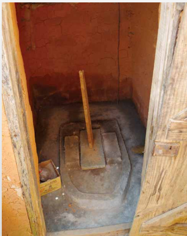
ABOVE LEFT: A FLY-PROOF LATRINE USING LOCAL MATERIALS AND BUILT AFTER TRIGGERING ACTIVITIES. CREDIT: WSSCC/DAVID TROUBA
